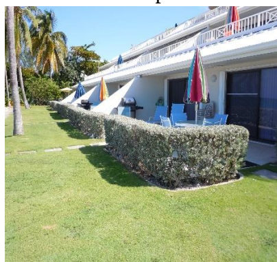
Ocean front metal roof and railings
