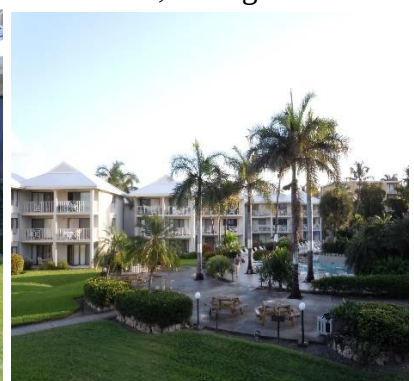
After major restoration
