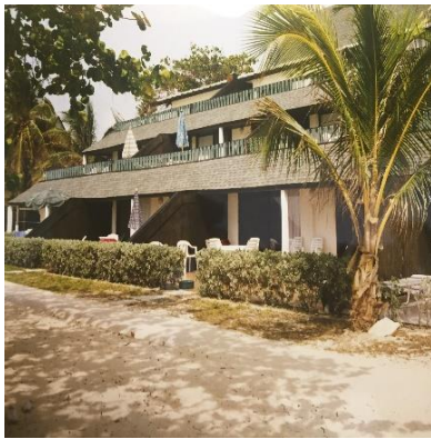
Ocean Front Asphalt Roofs
